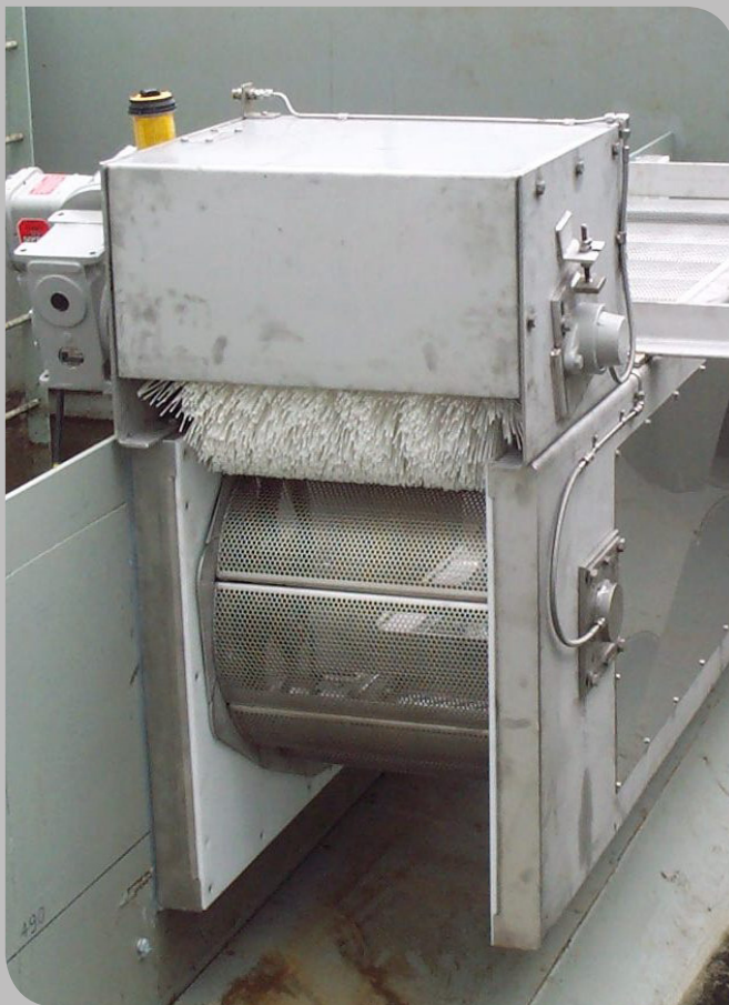
Figure 1 : StormGuard® Typical Installation
